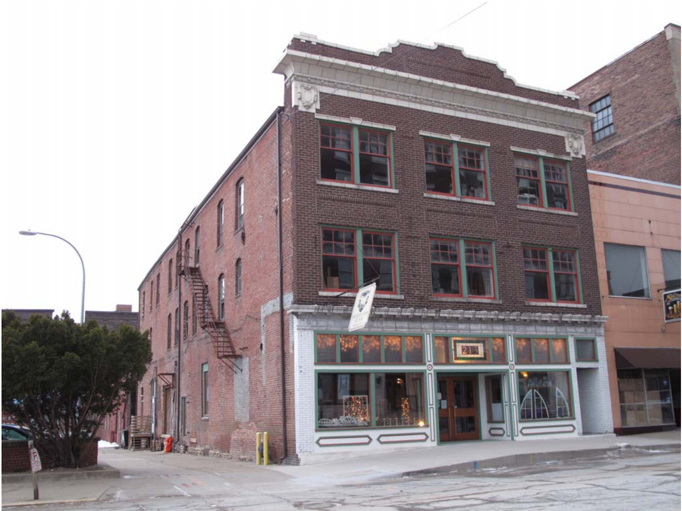
Photograph 29-01638-001 – North elevation, looking southwest (McCarley, January 14, 2014).
