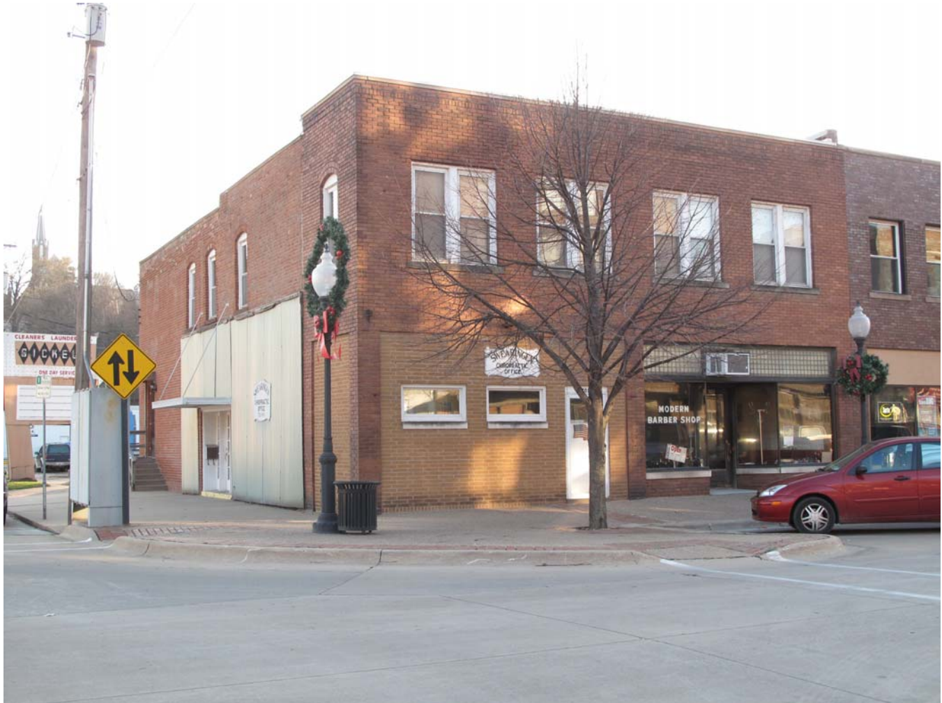
Photograph 29-03678-001 – East and north elevations, looking southwest (McCarley, November 15, 2012)
